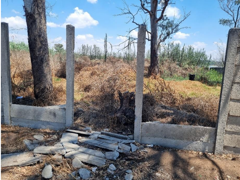
Damaged area of concrete slabs
